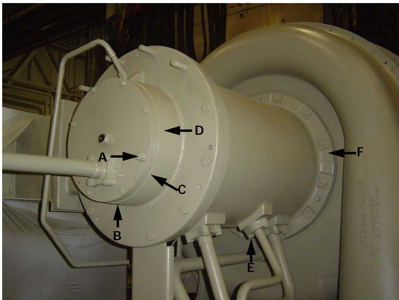
Figure 1. Recommended Vibration Data Collection Points
